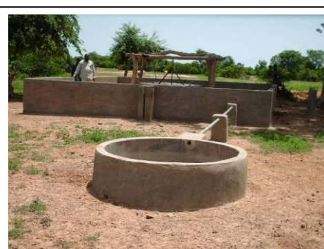
Photo 2: The Togouma pastoral well showing details of metal covering and the wall and concrete apron protecting the well surface from damage
