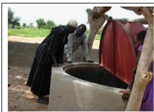
Photo 2: The Togouma pastoral well showing details of metal covering and the wall and concrete apron protecting the well surface from damage
